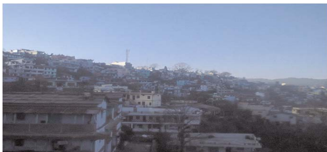
Plate-1 unplanned house constructions
